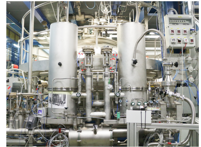
LXe purification system
